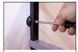
Using the appropriate hardware, install one of the lumber racks onto your wall. Each upright will use 3 spacers (part #6) each as shown in photo above. Secure the lumber racks. Note: Depending on what type of surface you are securing the rack to dictates what type of fastener to use. Included are standard wood screws for wooden wall mounting. Also included are bolts with anchors for cement wall mounting. See Parts Description Chart to determine which hardware to use.
